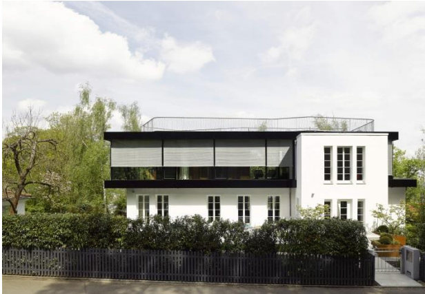
Picture 1: External, roll-up sun protection systems made from metallic mesh supplied by the company GKD protect the large, glazed second floor from overheating or undesirable insights.
