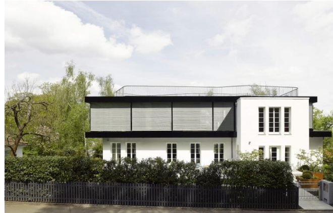
Picture 2: With their purist look, the metal roller blinds shimmer in the sunlight and underline the overall architectural concept.
