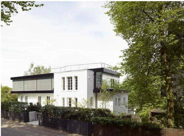
Picture 3: The chosen mesh type, Licorne 13A, has a normal-normal energy transmission level of just 0.2. That means 80 percent of the solar energy input is dissipated through reflection or diffusion.
