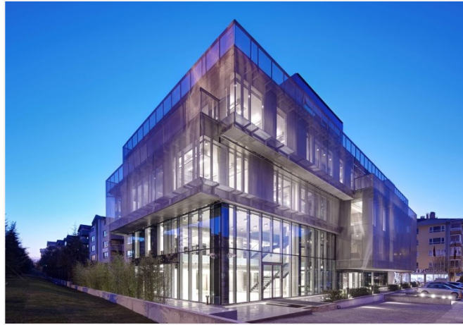
Picture 2: Solar protection façade made of Omega mesh at the new headquarters of the Turkish Contractors Association in Ankara.
