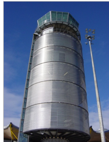
Picture 4: Madrid Barajas encapsulated two control towers with 1,600 square meters of ESCALE 7x1 stainless steel fabric from GKD.
