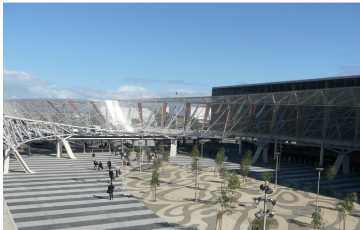
Picture 3: At Adelaide Airport in Australia, 2,000 square meters of TIGRIS stainless steel fabric from GKD were used for the extended and slanted façade of the path connecting the terminal with the parking garage.
