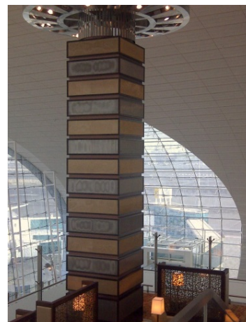
Picture 8: At Dubai International Airport, GKD metal fabric was used as cladding for the columns that stretch across multiple floors.
